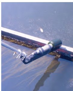
IFL with deflector for passing over a skimmer arm
