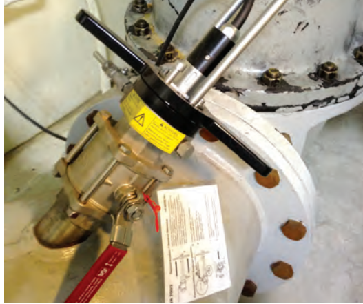
Pressurized, retractable insertion mount 2 bar or 10 bar overpressure
